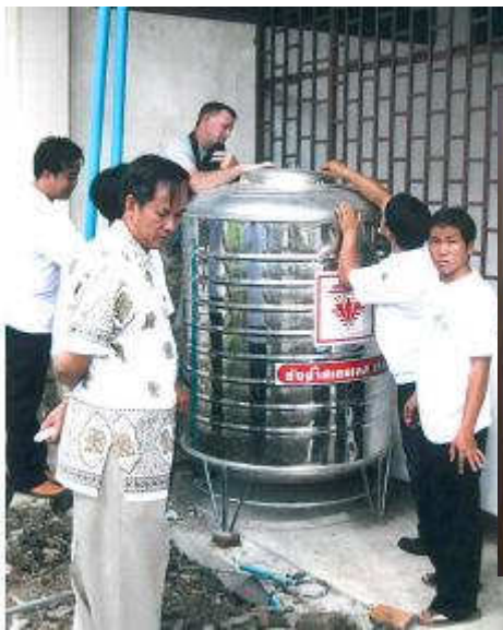
The 103 class installing the filtration system in Luang Prabang
